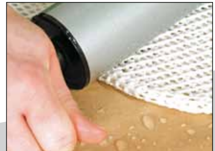
5. Heat areas to cut in water to soften and then cut.
